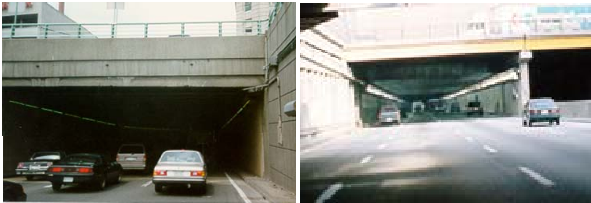
Figure 2-7 “Black Hole” (Left) and Proper Lighting (Right)
