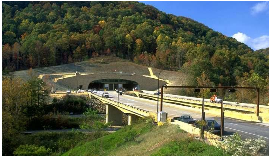
Figure 2-8 Portal Structure for Cumberland Gap Tunnel
